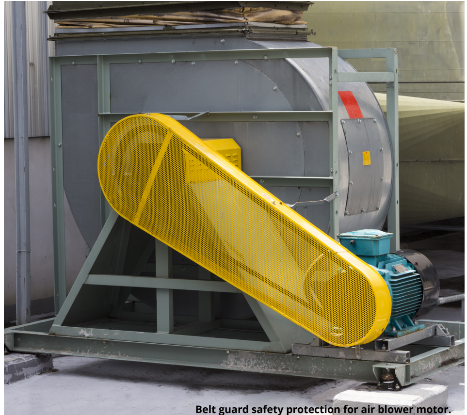
Belt guard safety protection for air blower motor.
