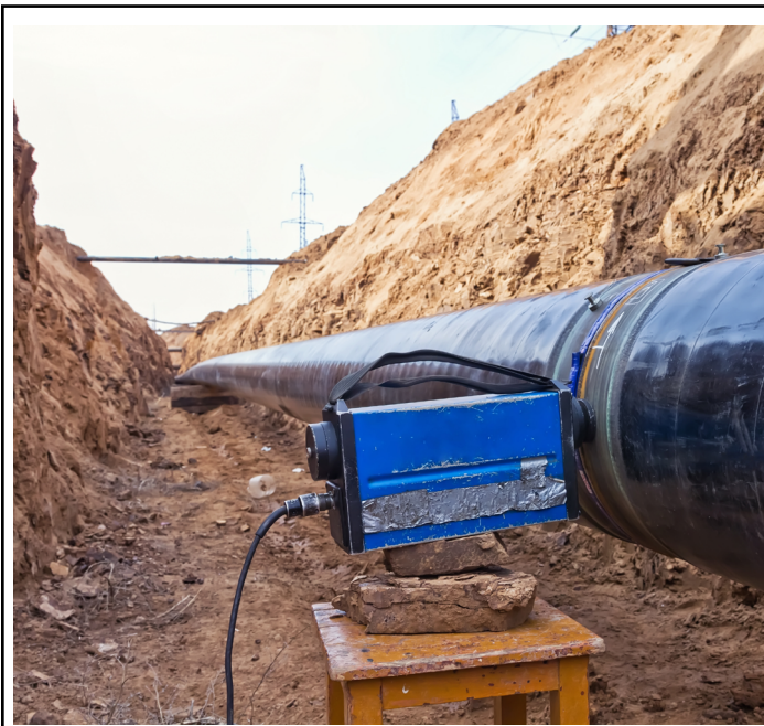
X-raying a pipeline's weld joints.
